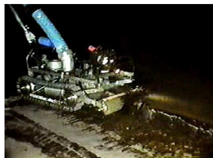
CST Machine "in action" cleaning
